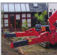
Level operation on uneven sites
